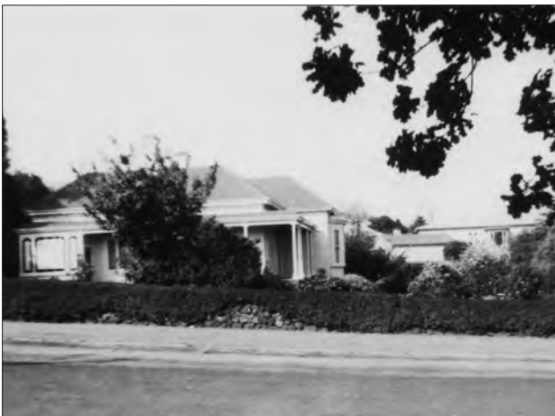
Brooks' villa at 25 Mt Albert Rd shortly before demolition in 1950s. Photo taken by Rich Afford.
